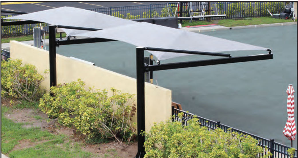
Pictured above are two new awnings at the lawn bowl courts. The previous awnings were damaged in a hurricane and had to be completely replaced.
